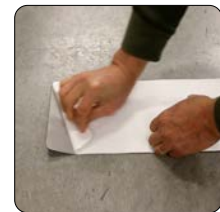
2) Peel. Begin to partially remove backing.
